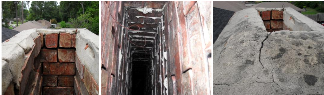
Missing mortar
