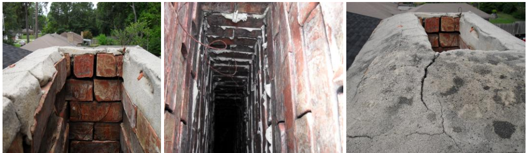
Missing mortar
